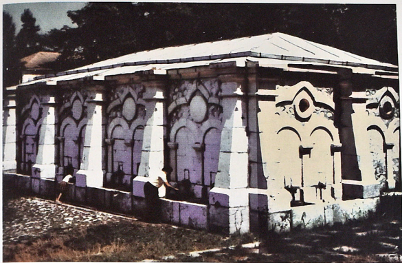
In 1872 Khurshid Banu Natavan ordered to construct the first water pipe in Shusha at her own expense. Water distribution points were installed in various districts of the city that started to be called bulags (springs) among people. In the picture you can see the main distribution point called "Khan gizi bulaghi".
