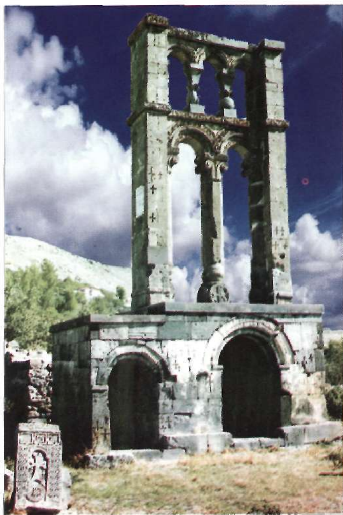
The look of Aghudi monument after the restoration.
