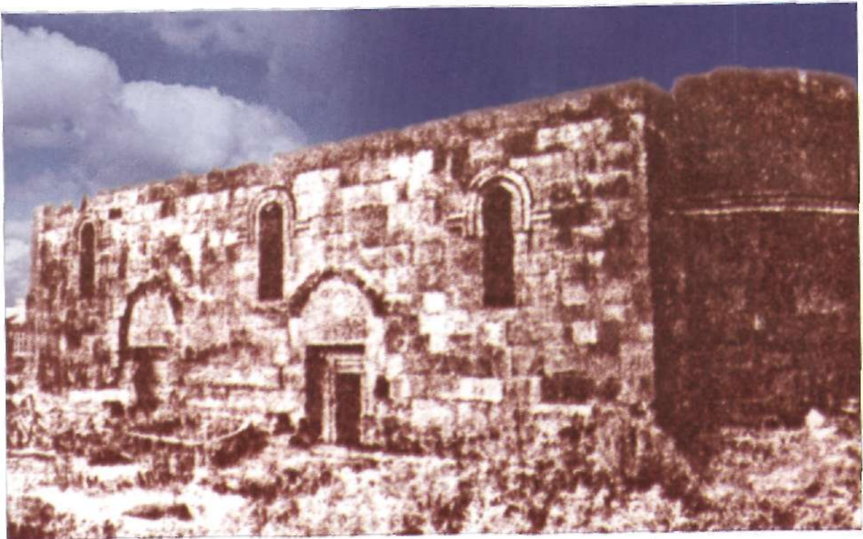
General view of Kasakh temple
