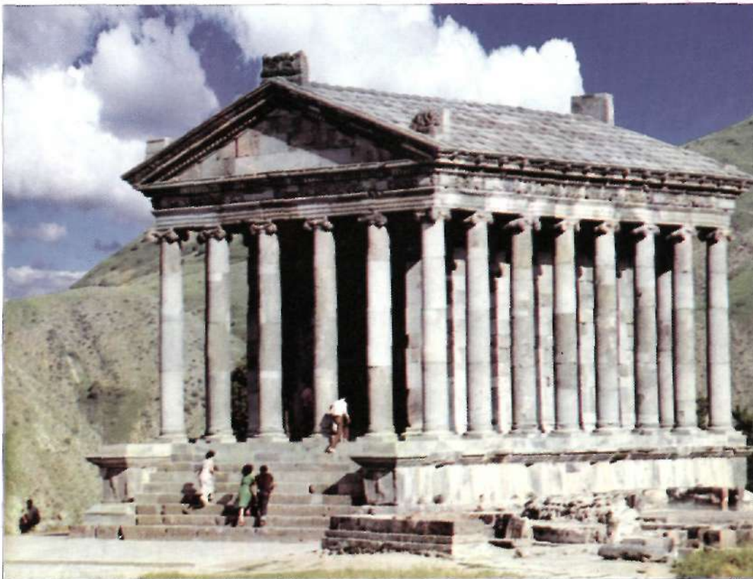
Garni temple after the restoration
