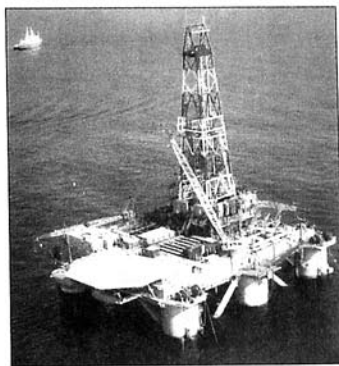
Semi-submerged drilling unit "Dada Gorgud", 1996
