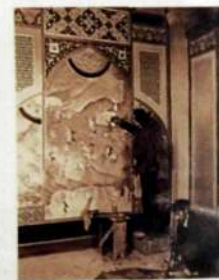
Restoration works in Saatly mosque
